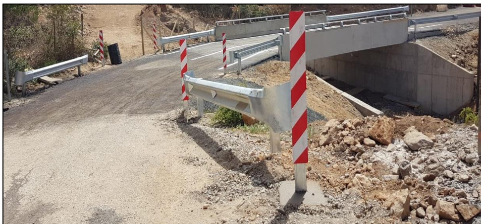
Figura 2.2.6 Baranda vehicular y peatonal
